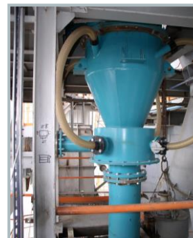
MULTIFLEX screw weigh feeder
